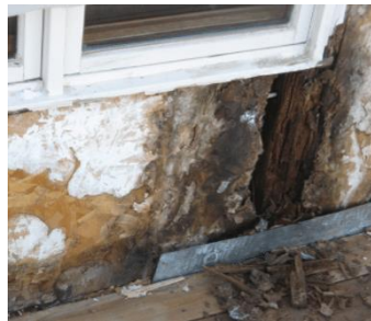
Figure 2: The EIFS wall became popular in the 90s and resulted in many moisture problems. Due to improper handling of rain water, moisture penetrated the wall and ended up trapped behind the exterior insulation.
