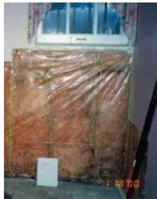
Figure 1: In warm/humid climate, an interior vapor retarder can cause intermediate condensation.
