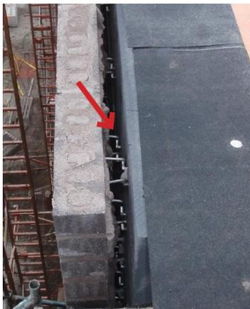
Figure 2: Typical rainscreen cavity at CMU wall with anchored masonry veneer
